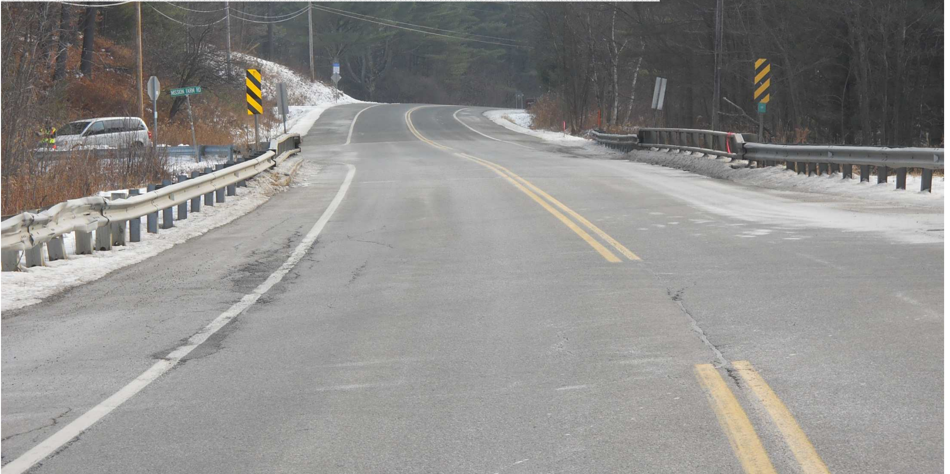
Bridge 33 Looking East
