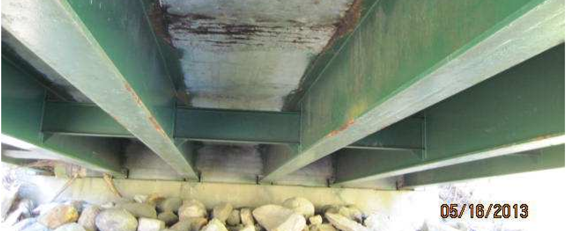
Typical deck deterioration with exposed rebar
