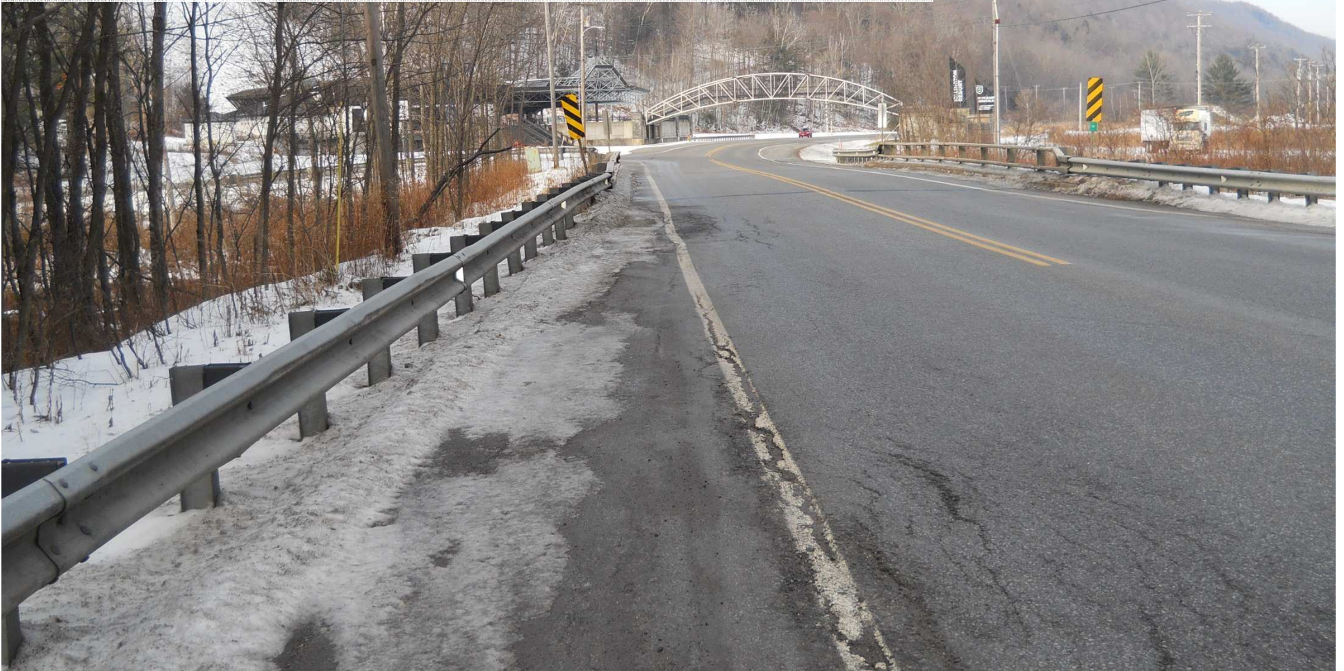
Bridge 33 Looking West
